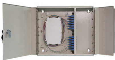
Storage of Spliced Fiber
